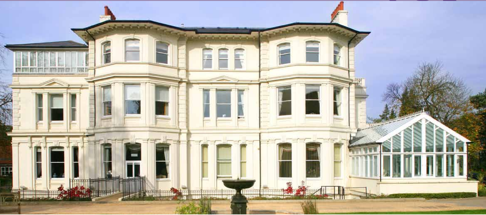
Willicombe Main House
